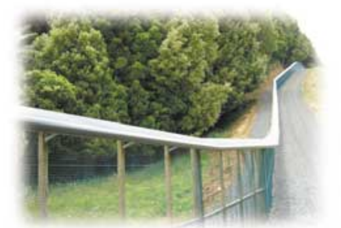
A section of the pest-proof fence along the south east bush line of the maunga.
